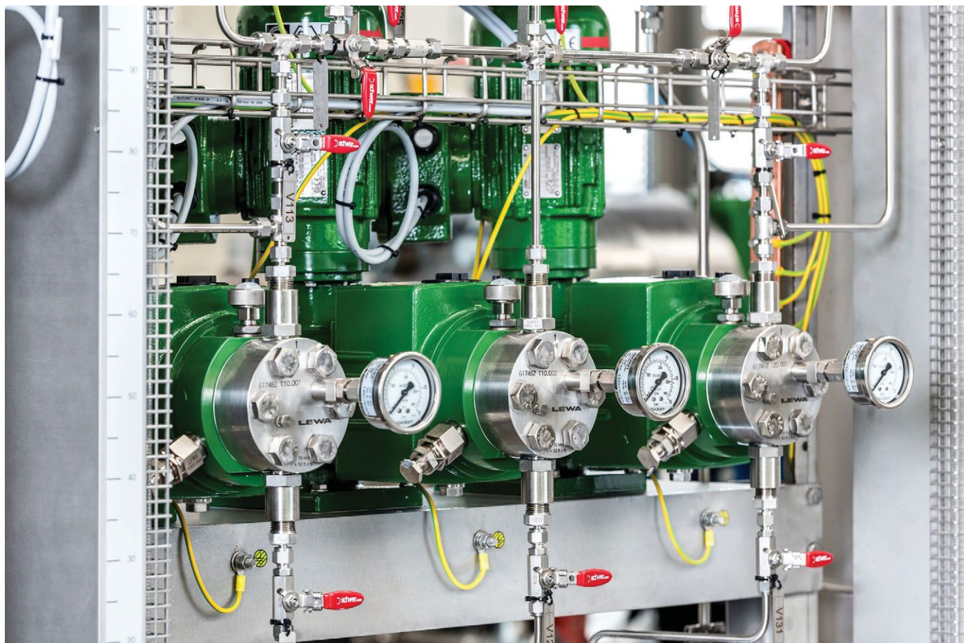
LEWA Smart Control guarantees metering accuracy. The controller handles this by carrying out a variance analysis and then instantly adjusting the flow rate as necessary.
