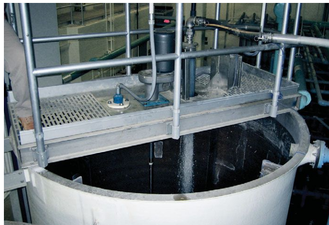
Many operational variables and characteristics must be considered before selecting a mixer. These include mixer type, fluid viscosity, rate of agitation, tank shape and volume, and pumping rate.
